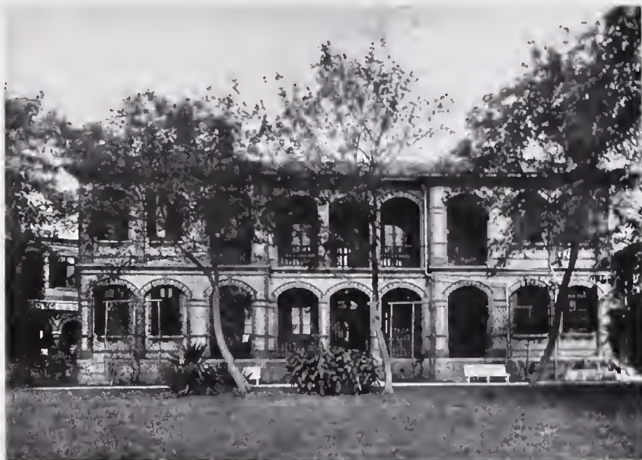
REAR OF WELLS WILLIAMS PAVILION
